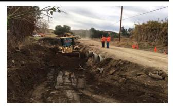
Work has begun on the water crossing at Margarth in the community of Good Hope to allow residents to be able to have a safer way out during the winter months and during flash floods. Work is expected to be completed within the next month for the crossing.
